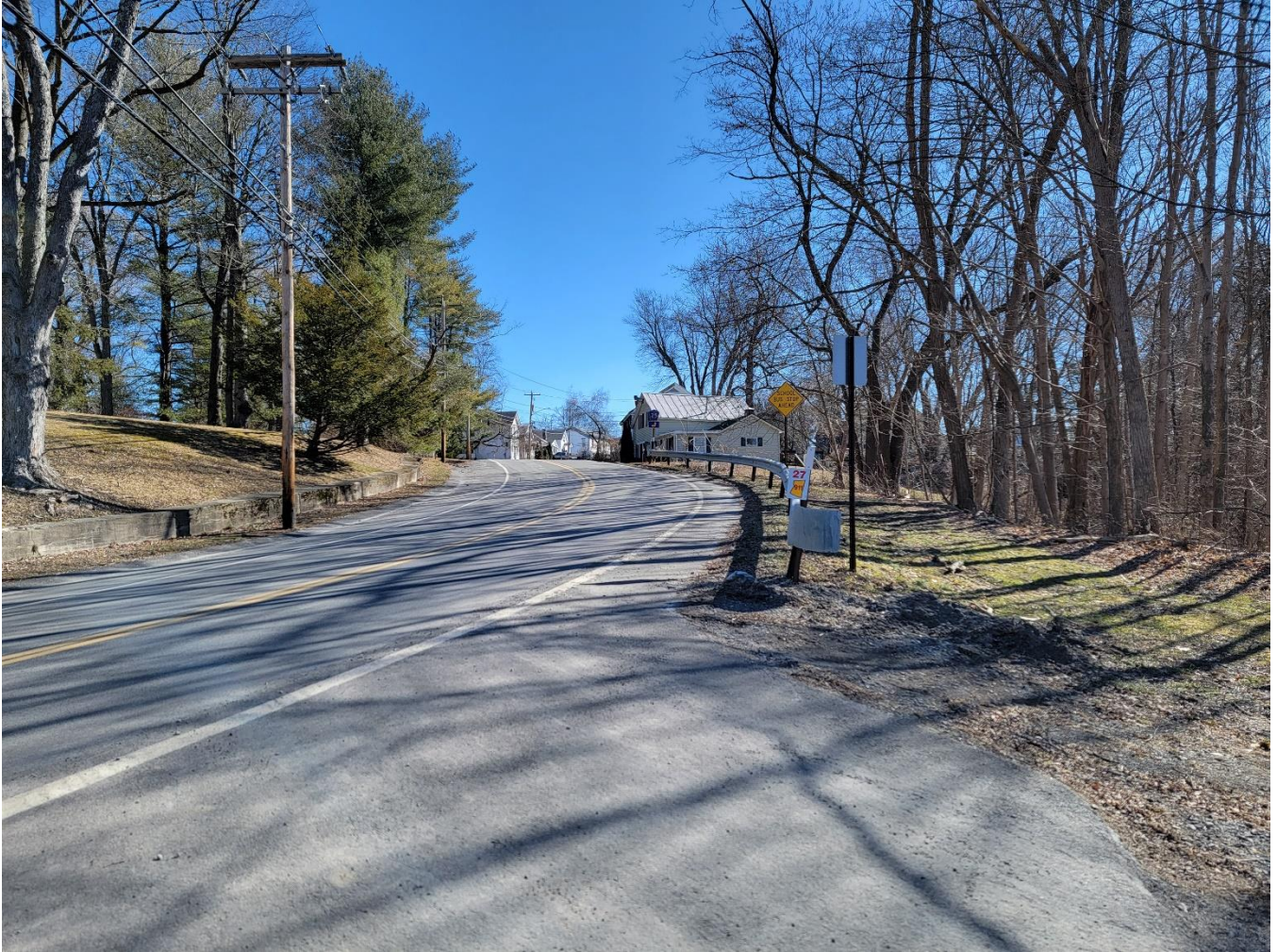
Photo 16: County Route 25A looking south adjacent to the Stuyvesant Falls Hydroelectric Station access road
