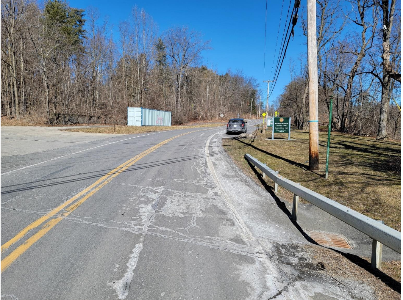
Photo 8: Looking north at the intersection of County Route 25A and New Street
