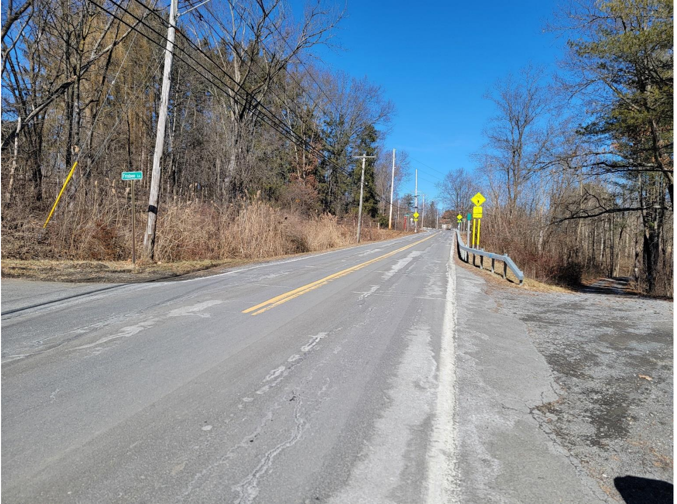
Photo 2: County Route 25A looking north adjacent to Frisbee Lane
