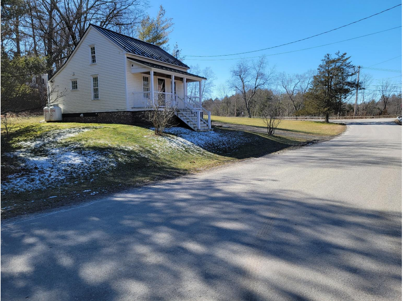
Photo 19: Lindenwald Avenue looking west at residential building (10 Lindenwald Avenue)
