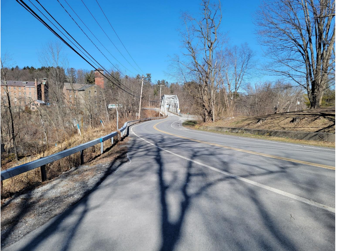
Photo 14: County Route 25A looking north near the Stuyvesant Falls Hydroelectric Station access road
